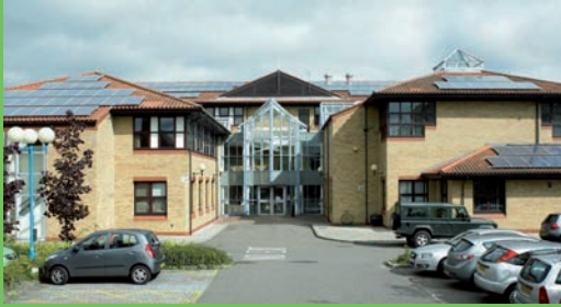
Council Offices 30 kWp
