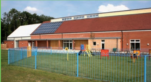
Community Centre 9.8 kWp
