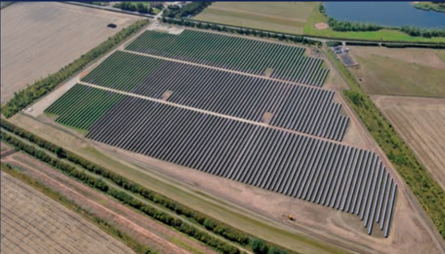
Lark Energy's 5MWp Solar Farm at Hawton, Newark
